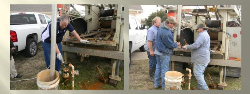
We rinsed the column down real well, then sealed off the bottom of the bailer and ran it up and down the column for 30 minutes to act as a surge block to push the Ultra C through the slots and into the gravel pack.
