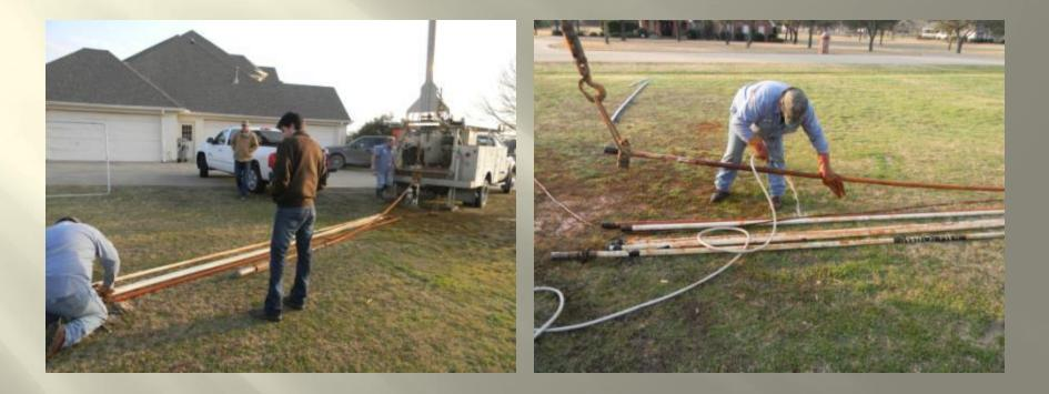
We arrived the next morning and started to put the pump and drop pipe back in. We rinsed off as much of the IRB from them as possible before we put them back in the hole.
