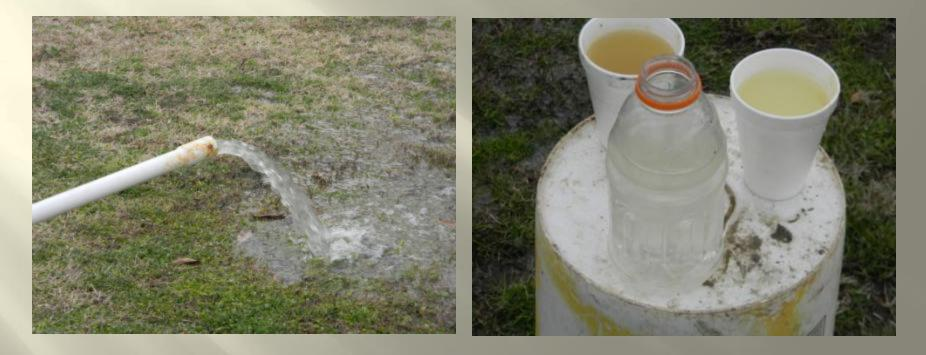
After surging for over 2 hours, we let the pump run untouched for one hour. After a total of 4 ½ hours pumping, the water was clear. This well had never had clear water before. The driller was so overcome, he bent down and drank some! He said he could still taste iron in it – but no one could see iron anymore.
