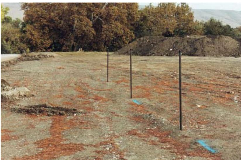
Always check for other underground utilities like gas lines or cables before pushing bars or rods into the ground over the pipe.
